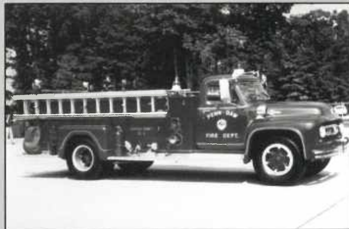
Penn Daw's 1953 Ford/Oren 750 gpm pumper was later converted into a light unit. Vienna, which owned a 1956 Ford, also had a similar conversion done on their pumper. (Mike Sanders photo).
